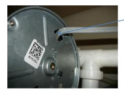
Electrical cord must pass through correct grommet.
